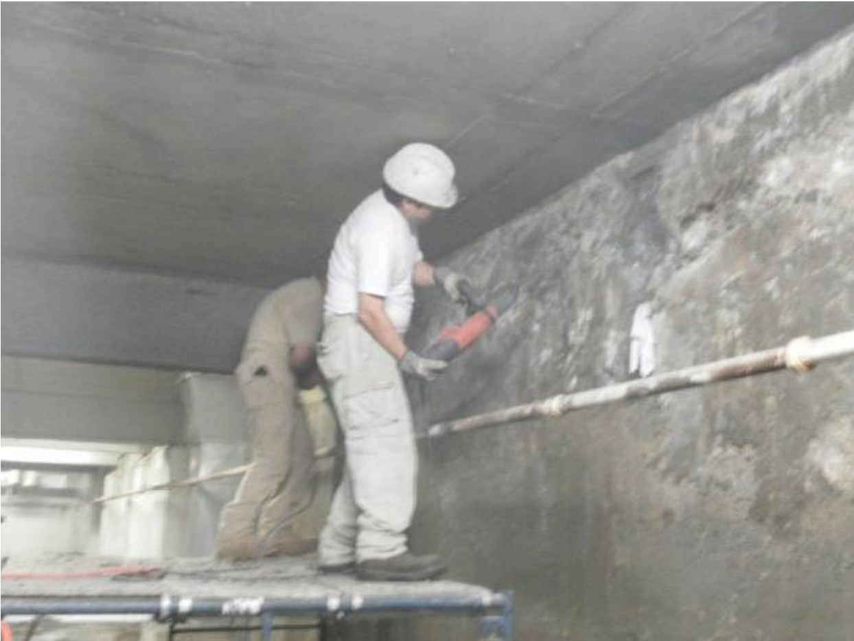
Bathurst – Waterproofing Foundation Wall Removing loose concrete and other contaminants
