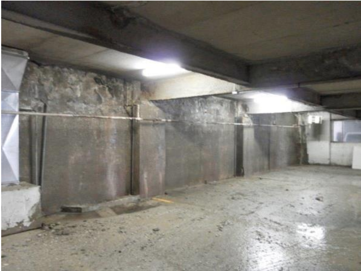
Bathurst – Waterproofing Foundation Wall Surface ready for application
