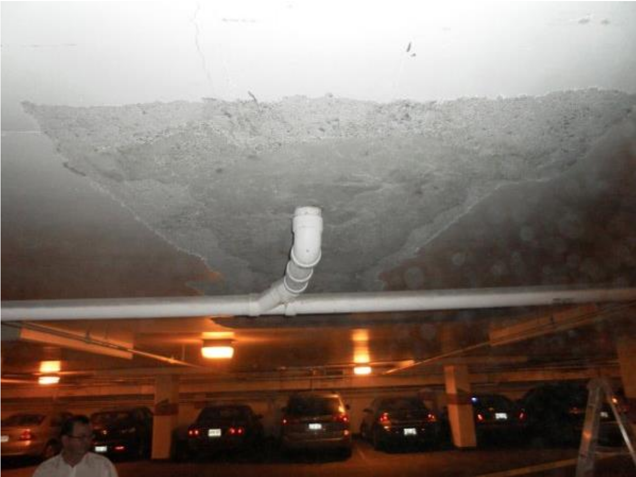
Carleton University underground parking garage waterproofing
