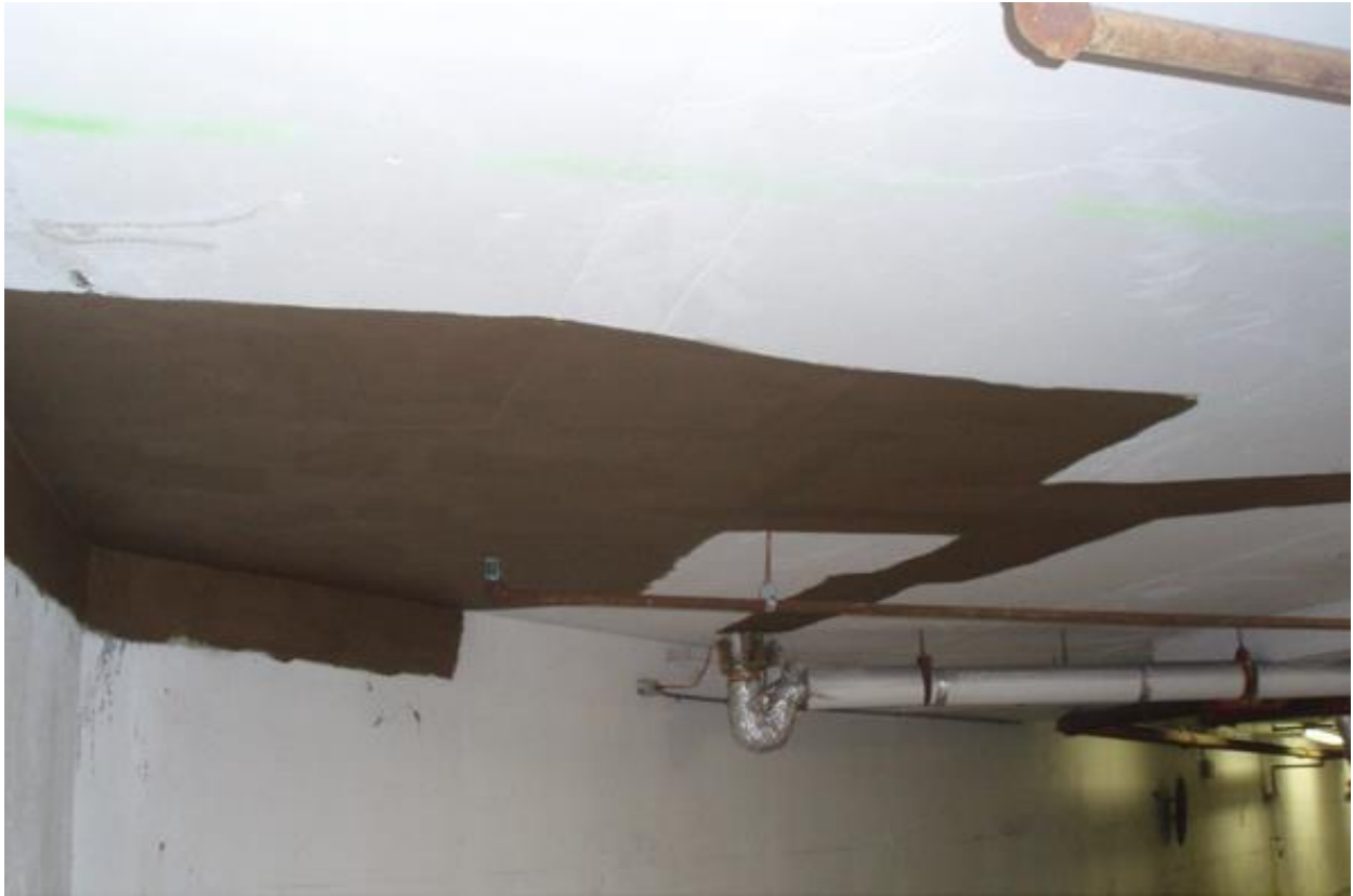
Ceiling slab waterproofing repair Final coat of CN2000C® and CN2000D®
