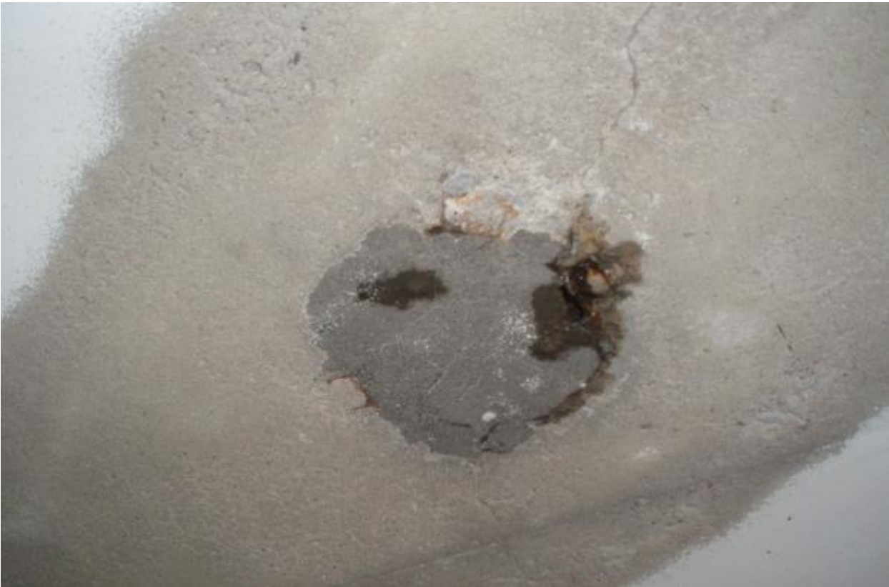
Ceiling slab waterproofing repair Point of seepage
