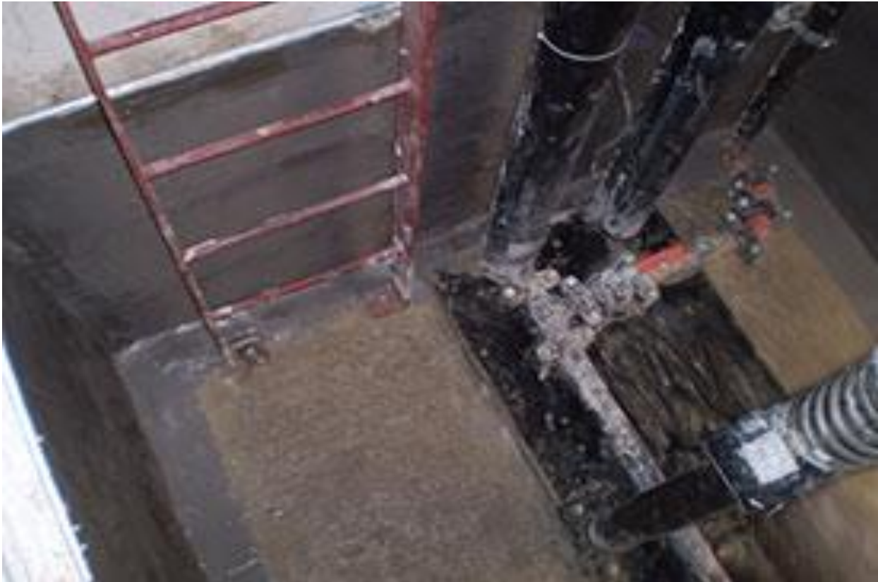
Commercial Building – Elevator pit
