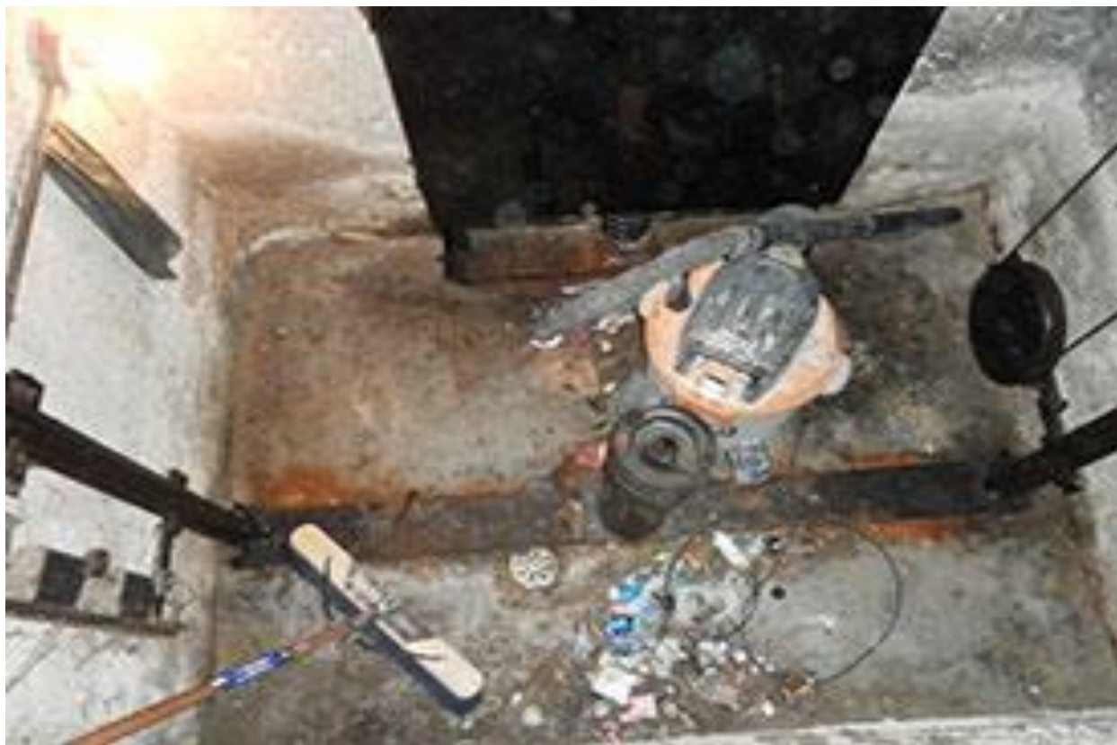
Condominium – Elevator pit
