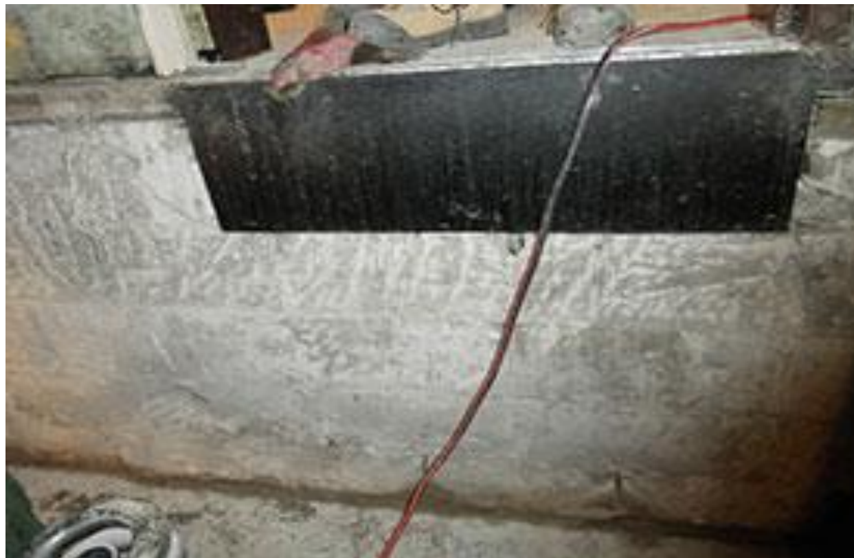
Condominium – Elevator pit
