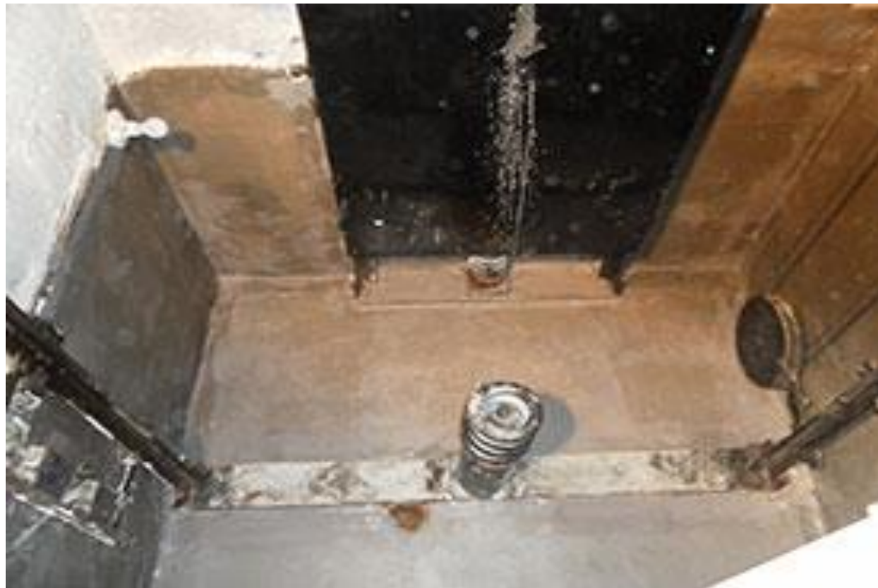
Condominium – Elevator pit
