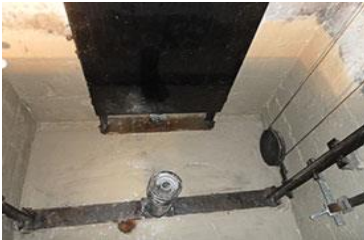
Condominium – Elevator pit
