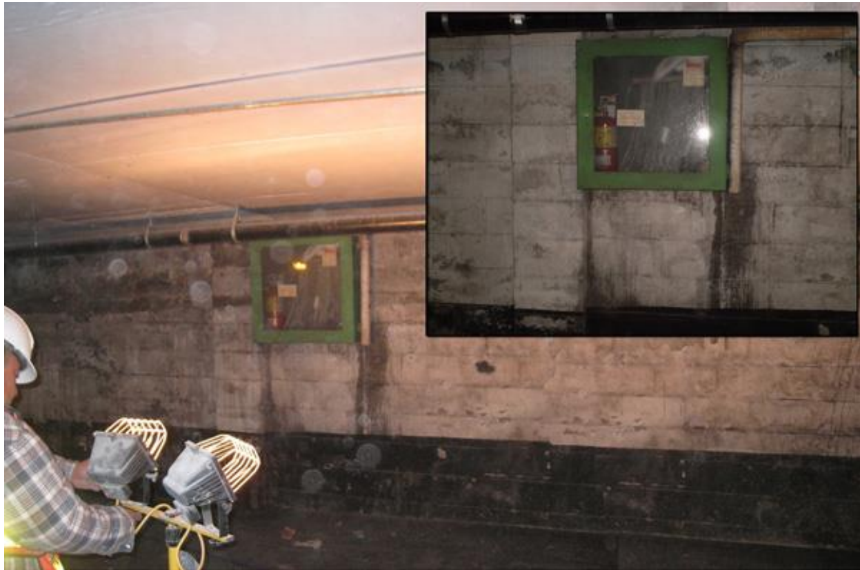
Lauder – Excavation not possible, below grade water infiltration Before
