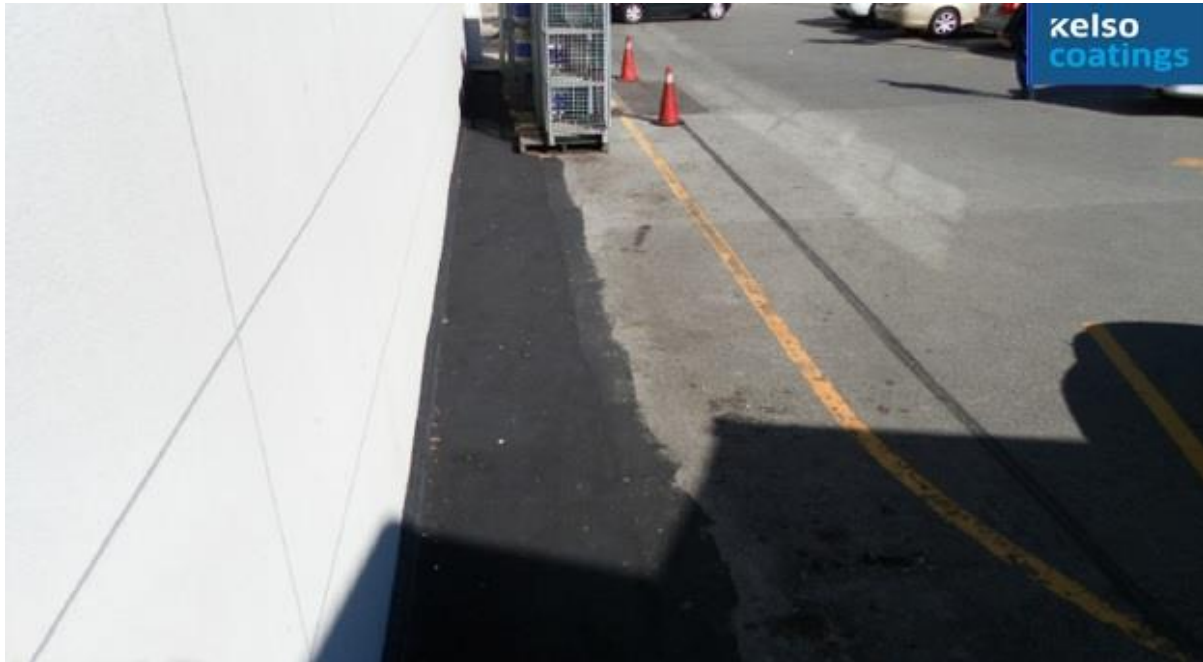
Canadian Tire, Toronto, Ontario Structural steel beams corroded due to water leakage
