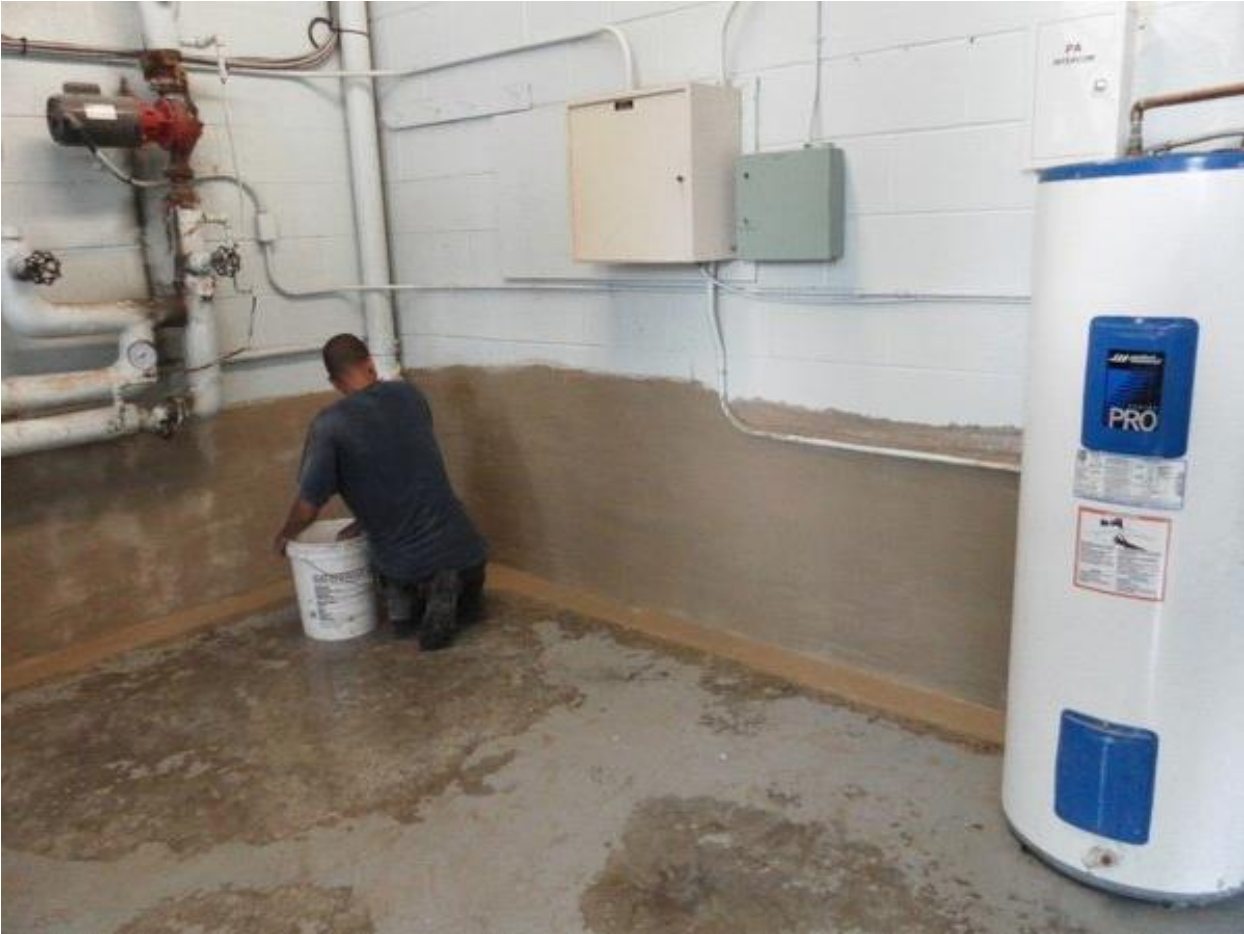
St John Bosco School boiler room waterproofing
