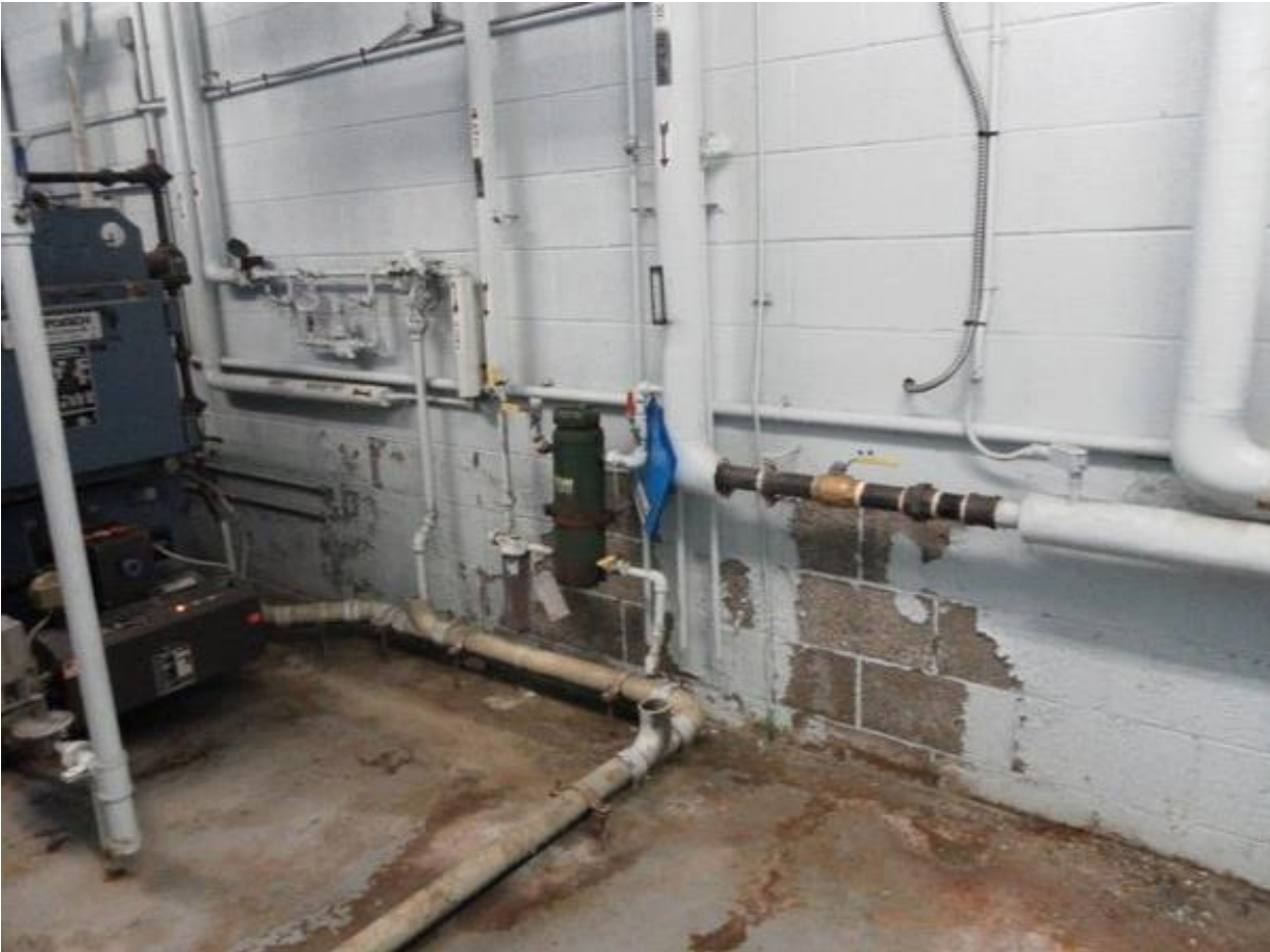
St John Bosco School boiler room waterproofing
