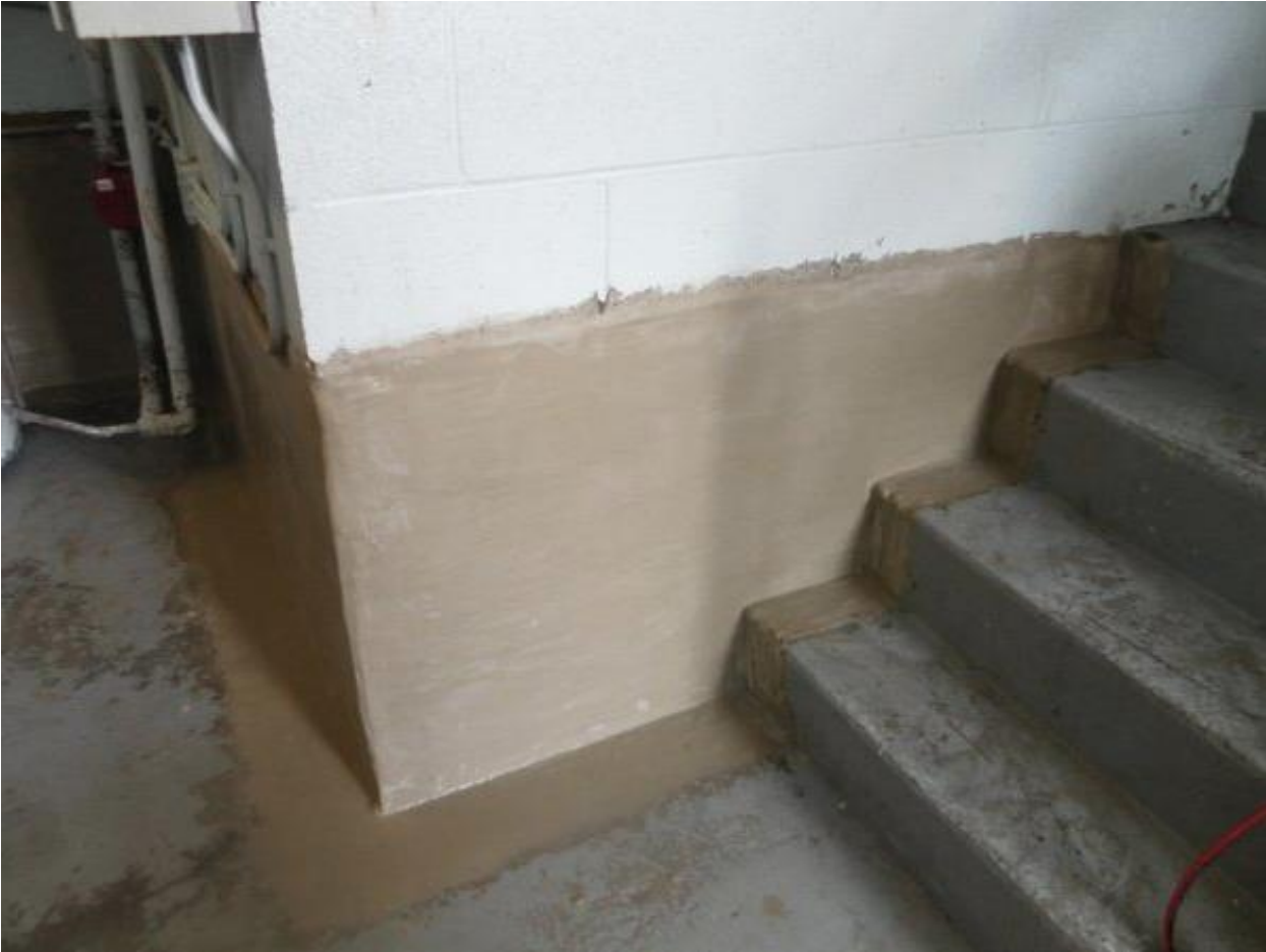
St John Bosco School boiler room waterproofing
