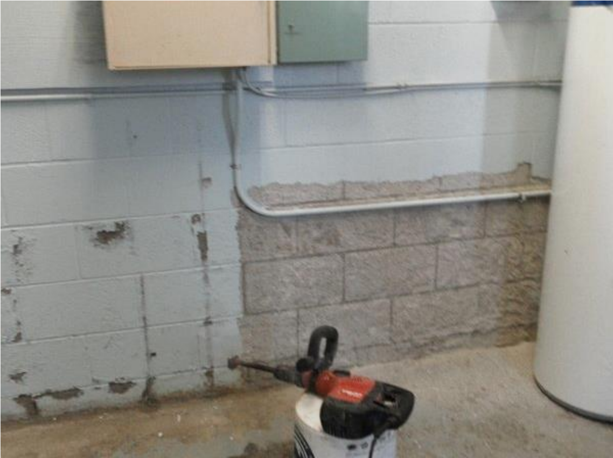
St John Bosco School boiler room waterproofing
