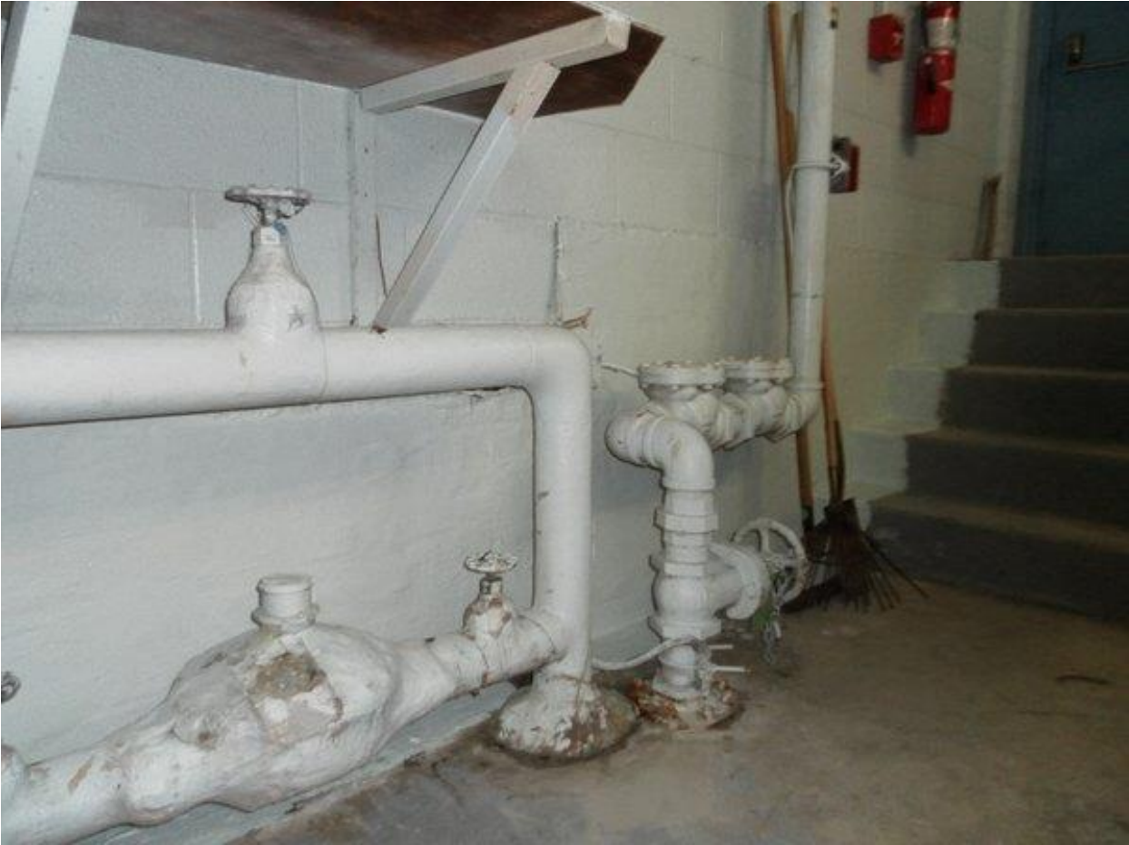
St John Bosco School boiler room waterproofing
