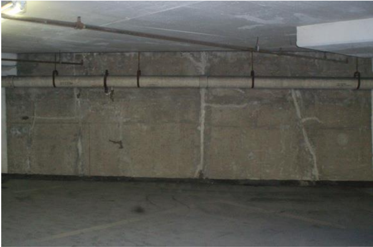
Townsgate – Foundation wall waterproofing Kelso team chased the cracks
