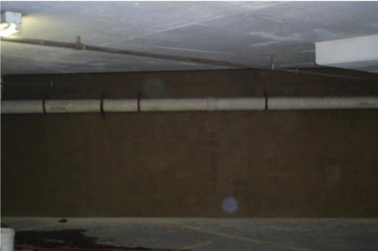
Townsgate – Foundation wall waterproofing Final coat of CN2000B®
