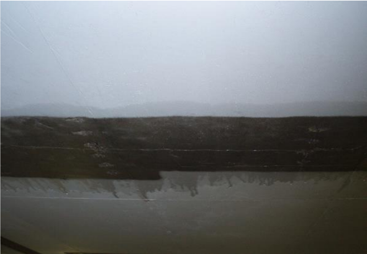
Townsgate – Parking ramp
