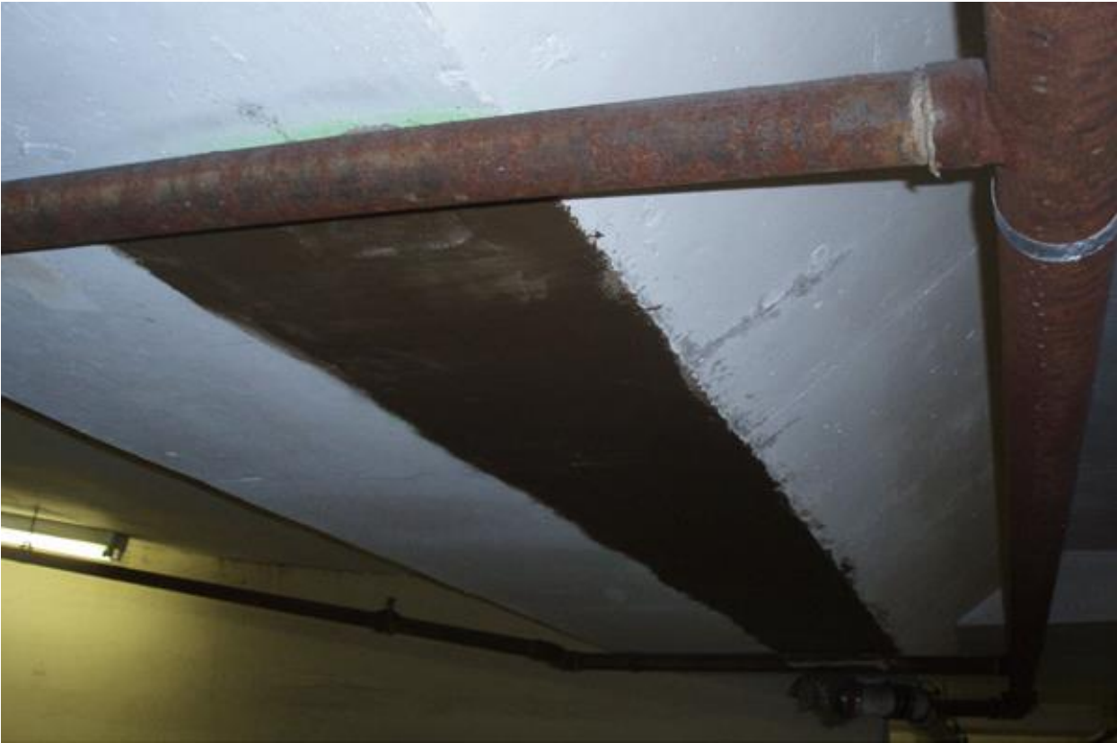
Townsgate – Parking ramp
