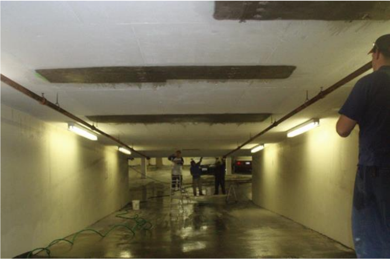
Townsgate – Parking ramp
