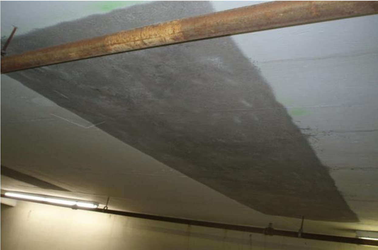
Townsgate – Parking ramp
