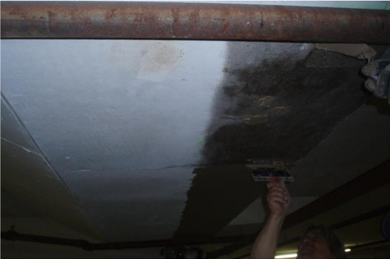
Townsgate – Parking ramp
