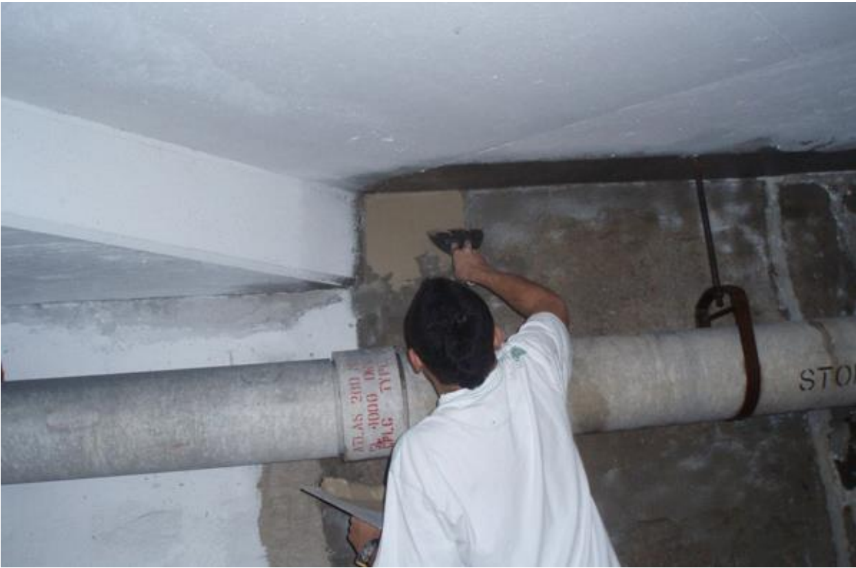
Townsgate – Y pipe
