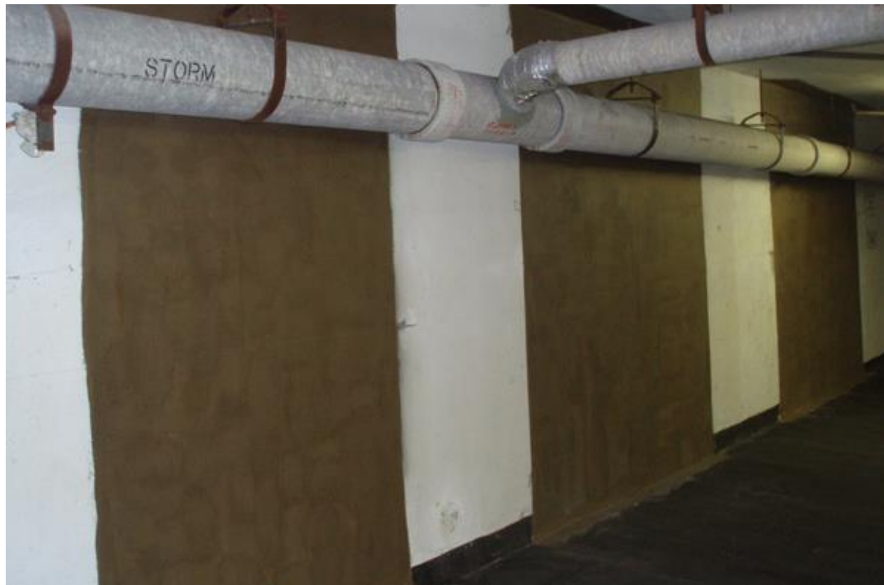
Townsgate – Y pipe
