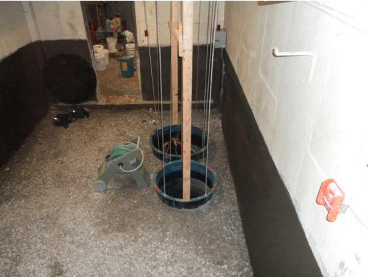
Warren Park below grade foundation wall waterproofing
