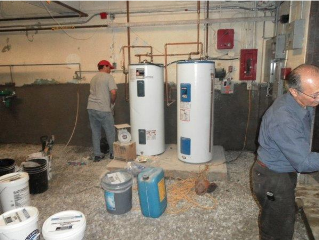
Warren Park below grade foundation wall waterproofing
