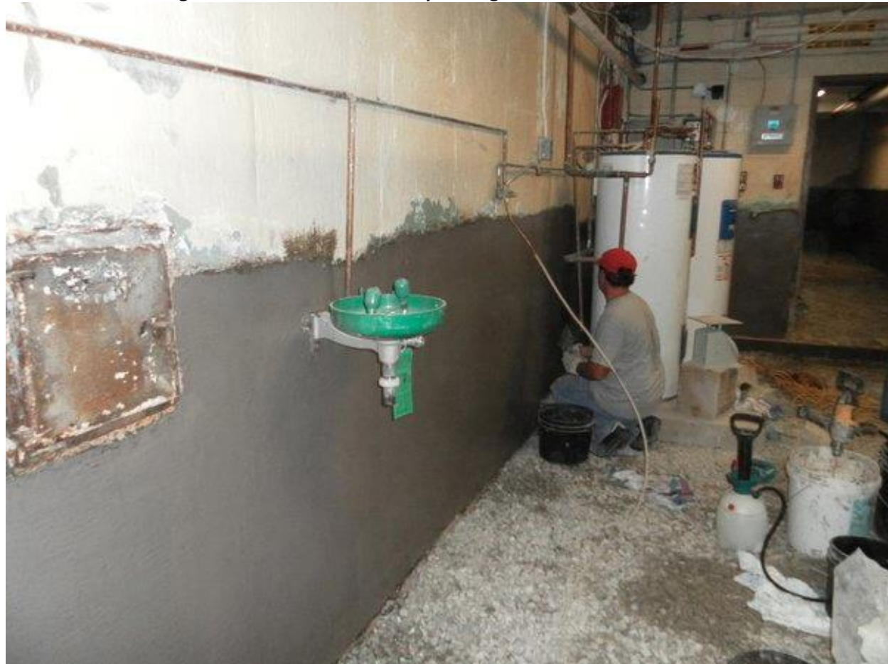
Warren Park below grade foundation wall waterproofing
