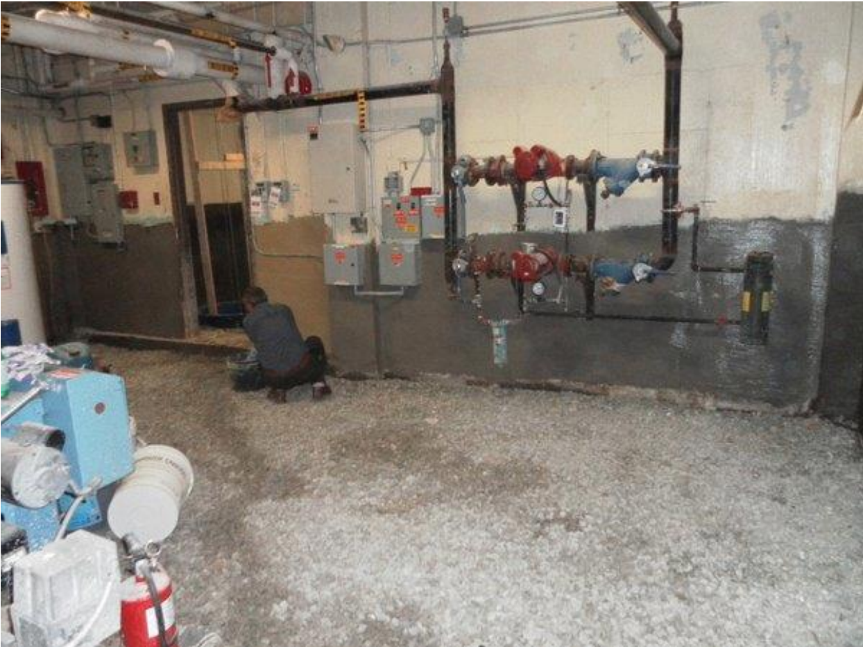
Warren Park below grade foundation wall waterproofing
