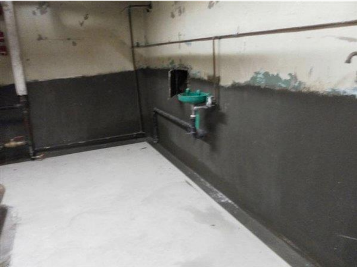
Warren Park below grade foundation wall waterproofing
