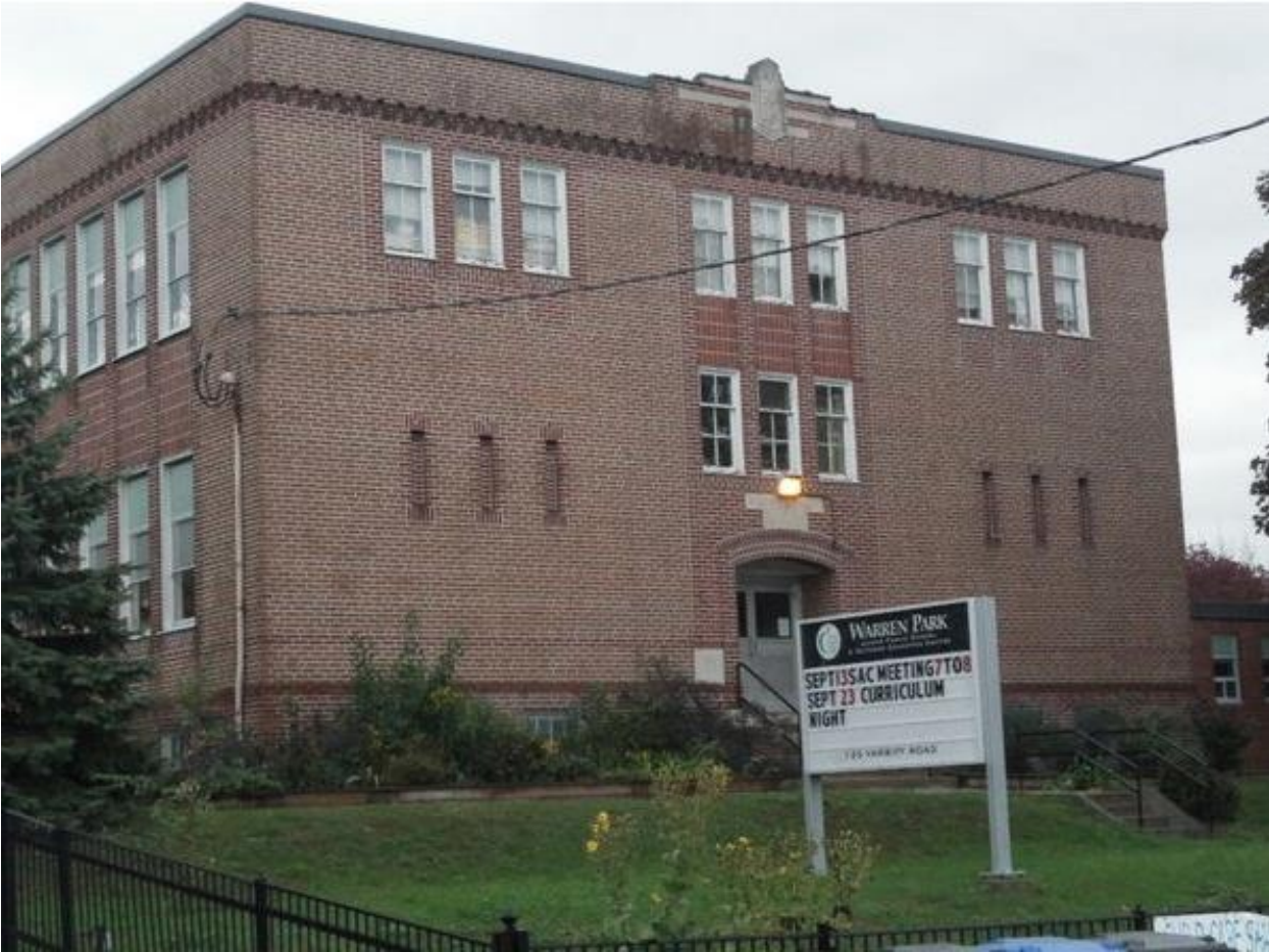
Warren Park below grade foundation wall waterproofing
