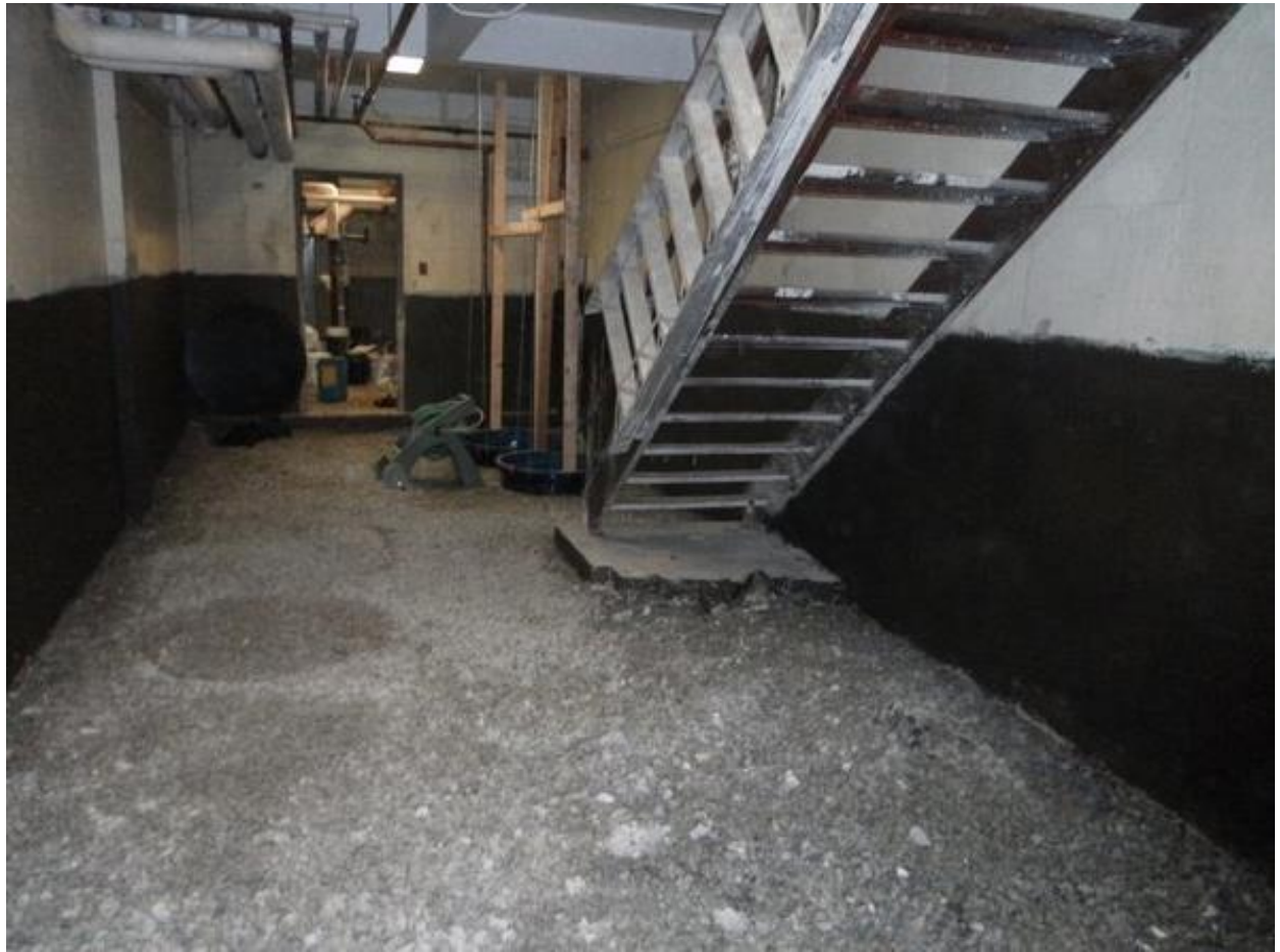
Warren Park below grade foundation wall waterproofing
