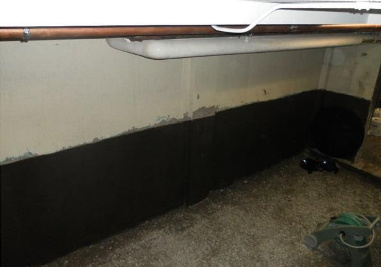
Warren Park below grade foundation wall waterproofing
