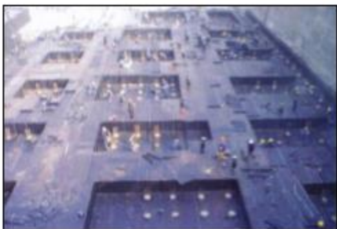
Figure 3 - “Water Cube” pile foundation site
