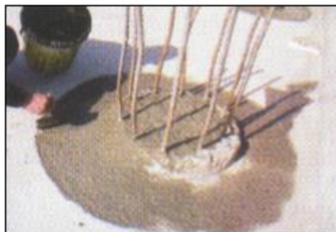
Figure 4 - Brush coating piles head with CN2000 waterproofing material
